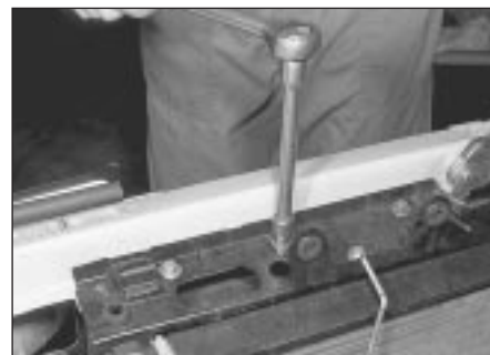
3.4a Undoing radiator retaining bolts
