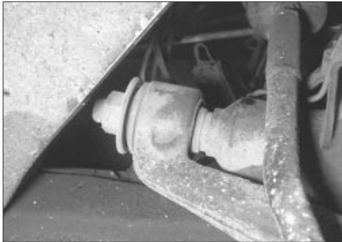
27.3 Check each rubber bush for splits, cracks or contamination of the rubber
